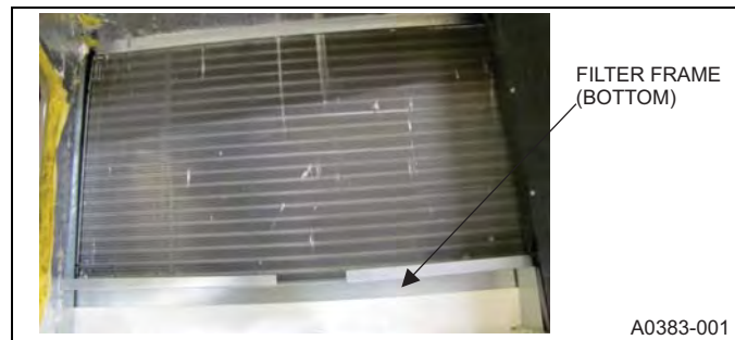
FIGURE 3: Filter Frame in Mounting Position.
